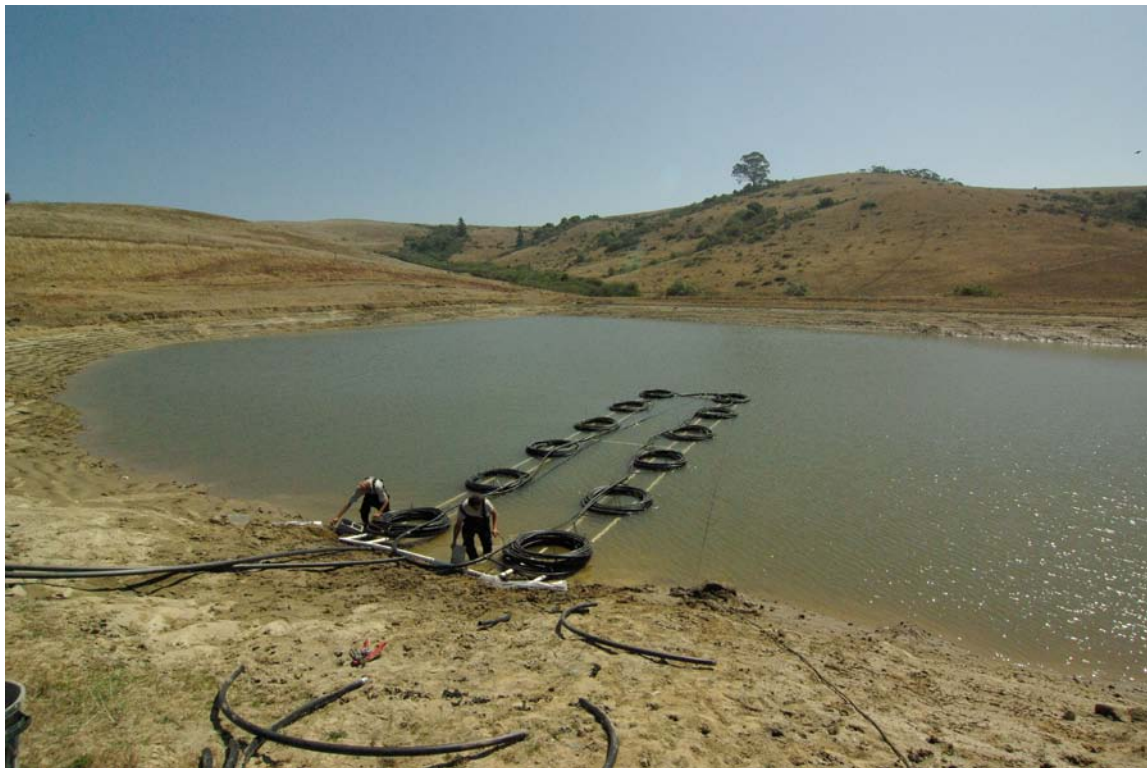
Figure 22: Example of pond loop prior to submergence
