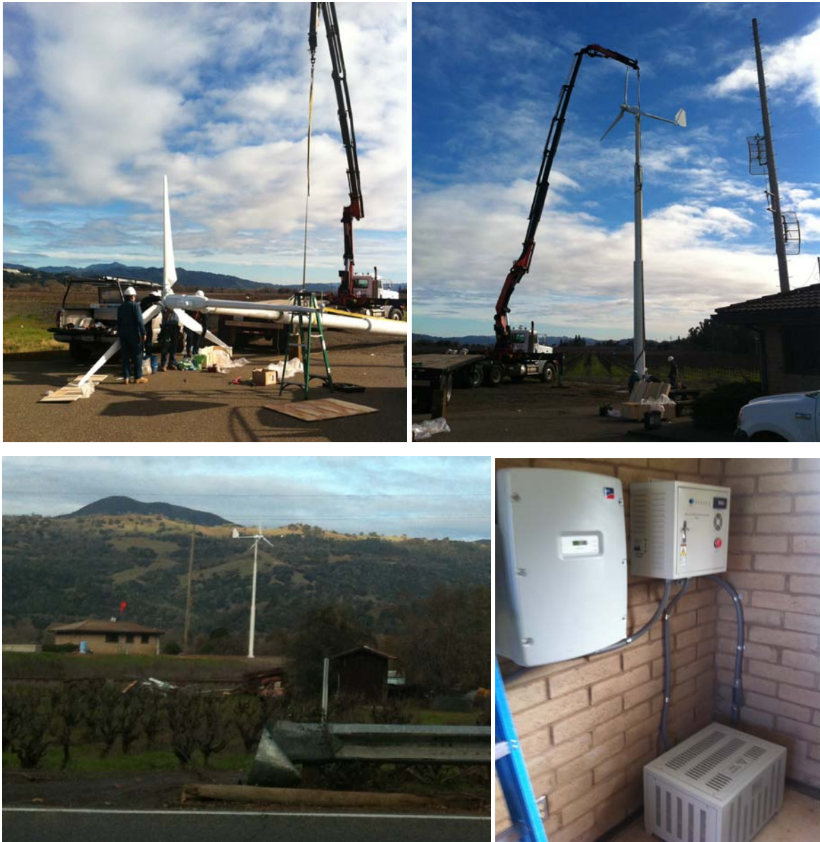
Figure 18: Wind turbine assembly and installation
