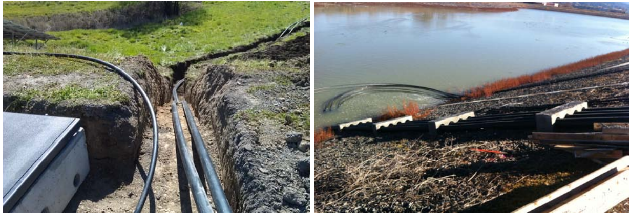
Figure 21: Pond loop trenching concrete pipe guides
