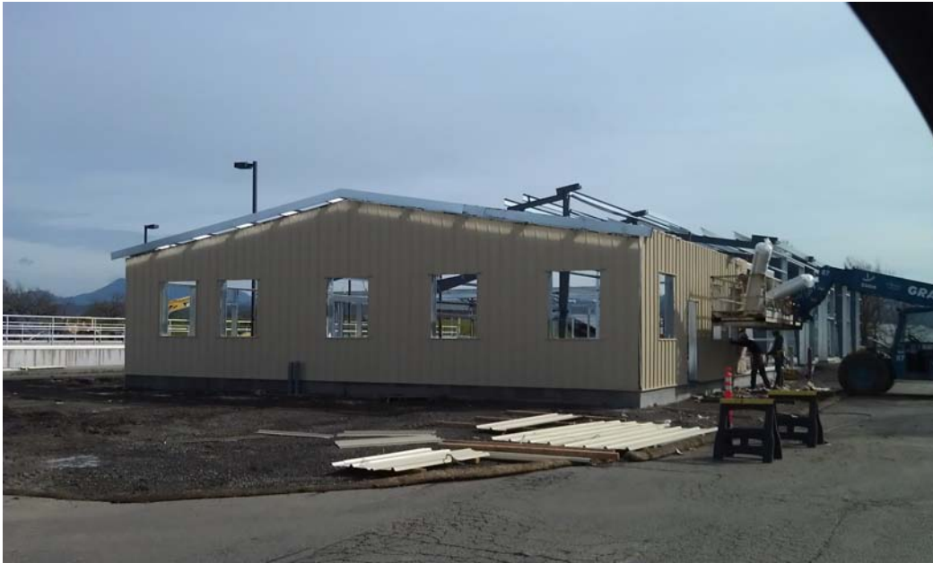
Figure 19: ALWSZ new Service Center construction
